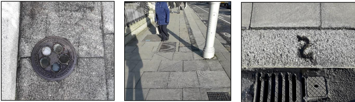
Figure A1.15: Historic Street Furniture on St Stephen's Green East: Coal Hole Cover (Nos 39-40), original Granite kerblines retained towards path centre (Nos 39-45) and probable Mason's Mark (No. 55)
