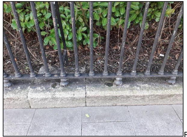
Figure A1.6: Visual survey of railings on St Stephen's Green East (A: railings with deteriorated paint. B: rust on horizontal rail scarf joint. C: missing spear head finials. D: failure of lead fixing, note chipped and weathered plinth. E: evidence of previous rearrangement of railings (empty sockets), flushed mortar and chipped and weathered plinth.
