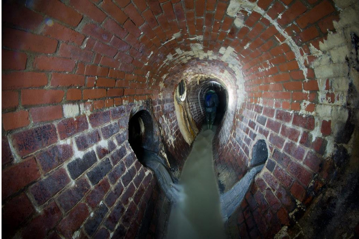
Figure 4.5: Typical Victorian Brick Sewer
