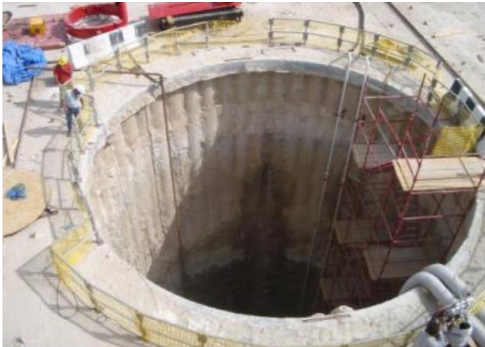
Figure 4.4: Intervention Shaft being Constructed by Secant Pilling Method
