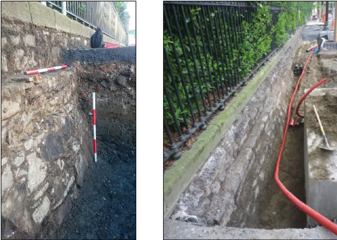
Figure 2.5: Images of the revetment wall of the perimeter ditch as it relates to the present day railings and plinth of the park's perimeter boundary (RPS 7751). Identified on St Stephen's Green North (Rubicon Heritage Ltd.)
